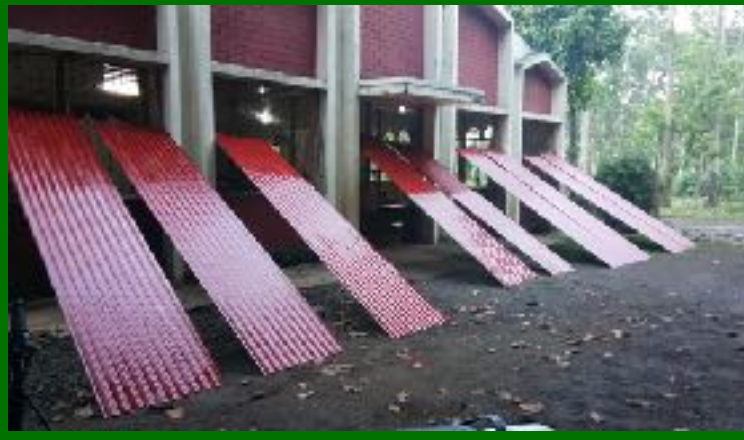
Providing new roofing for the church
